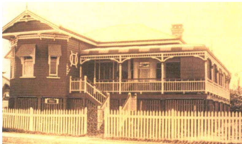
Belvedere, Florence Street, still standing today
