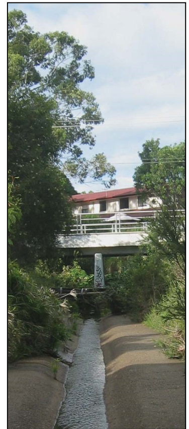
Tingal Road Bridge over Wynnum Creek. Circa 2003.
