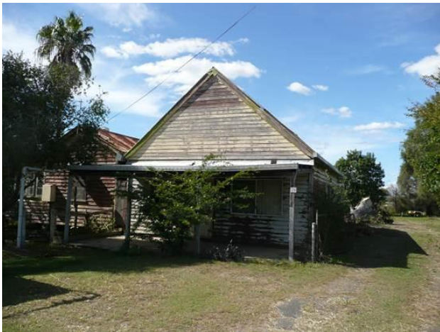
Prior to renovation
