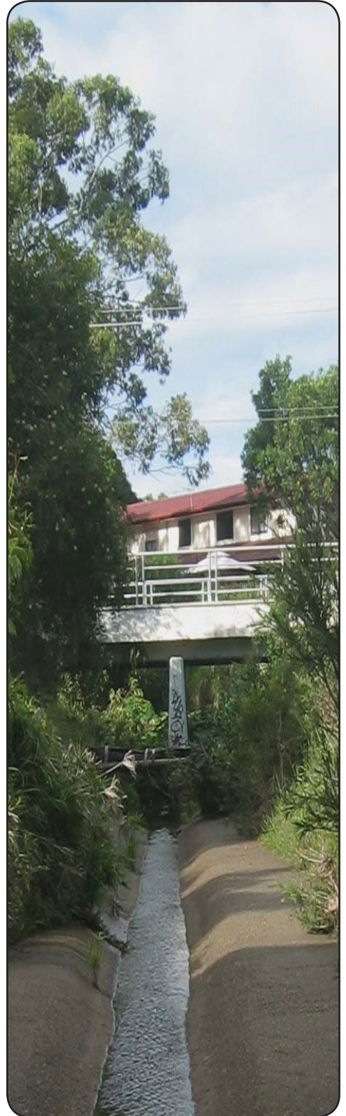
Tingal Road Bridge, Wynnum Creek. circa 2003
