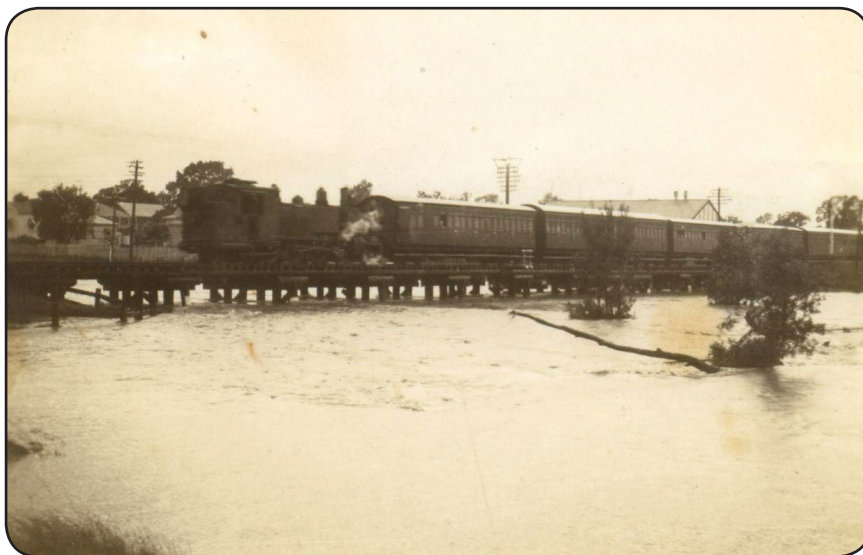
Tingal Road, Rail line. Flood 1974
