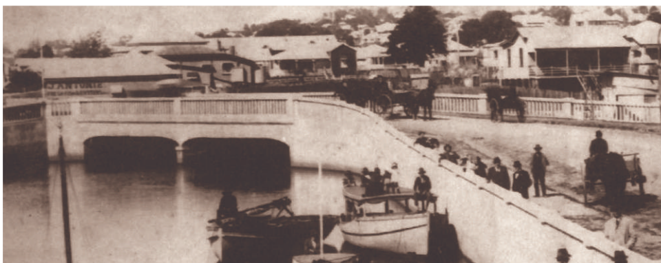
'Wynnnum Bridge', at the time of its opening in 1921.
