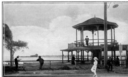
No. 2 JETTY, WYNNUM SOUTH
