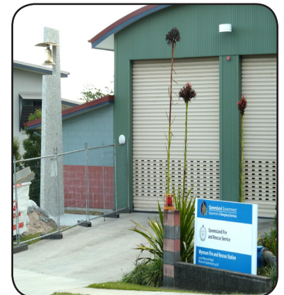
Wynnum Fire and Emergency Station August 2014
