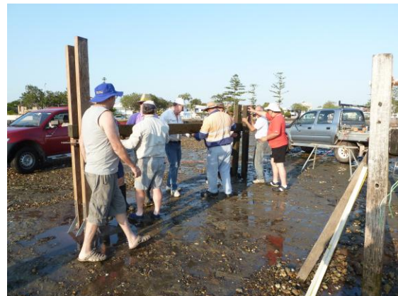
7.00 am – almost complete.
