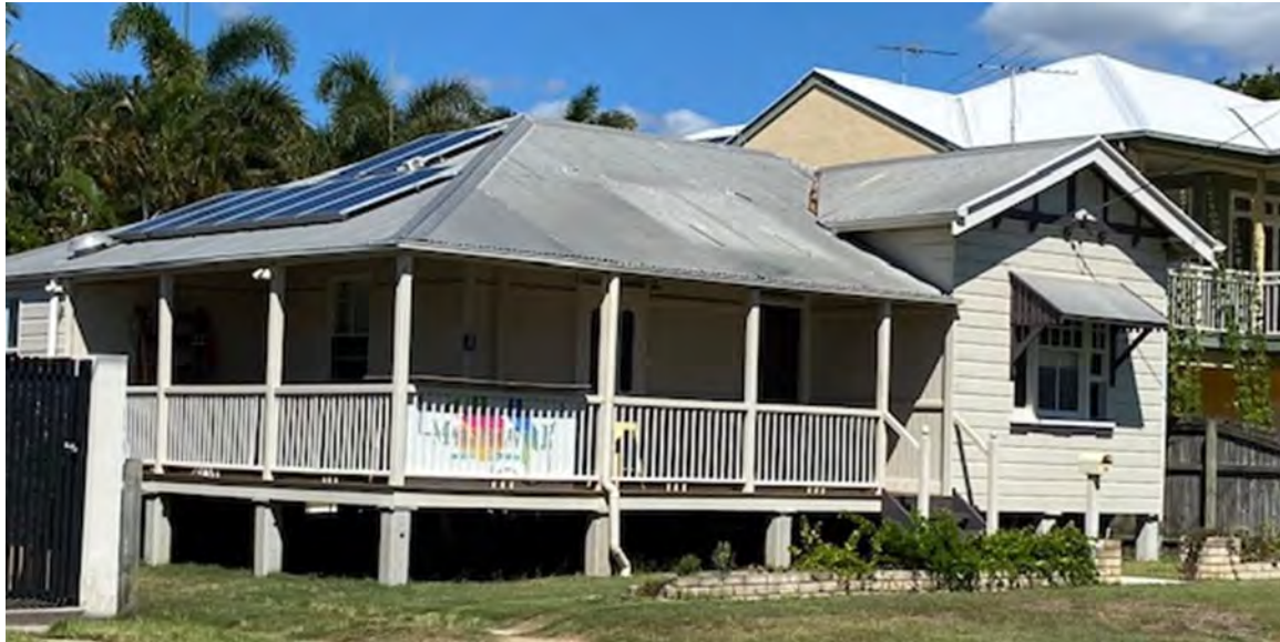
Asymmetrical Bungalow with L-shaped verandah – Alkoomie Street, Wynnum. Pre-1916.
