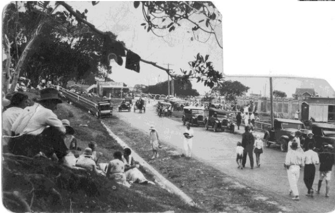
The walls and steps would have been built during the late 1920's to 1930's during the Great Depression, under the relief Work Scheme introduced for unemployed persons. The State paid the wages and the Local Authority fund the tools and the materials.
