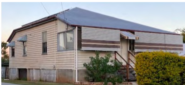
The house today at 201 Wynnum North road
