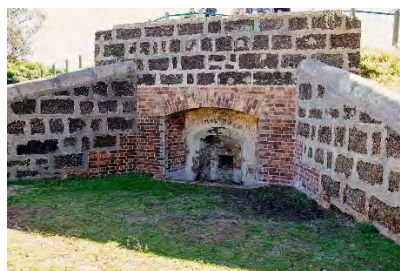
St Helena Lime Kiln was built in 1869 by prisoners. Image courtesy Amanda Thepanda.
