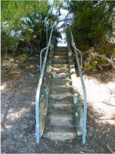
Steps leading to the top of Roles Hill Reservoir No.1
