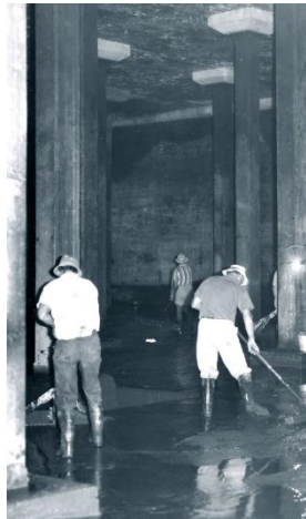
Inside Roles Hill Reservoir No. 1
