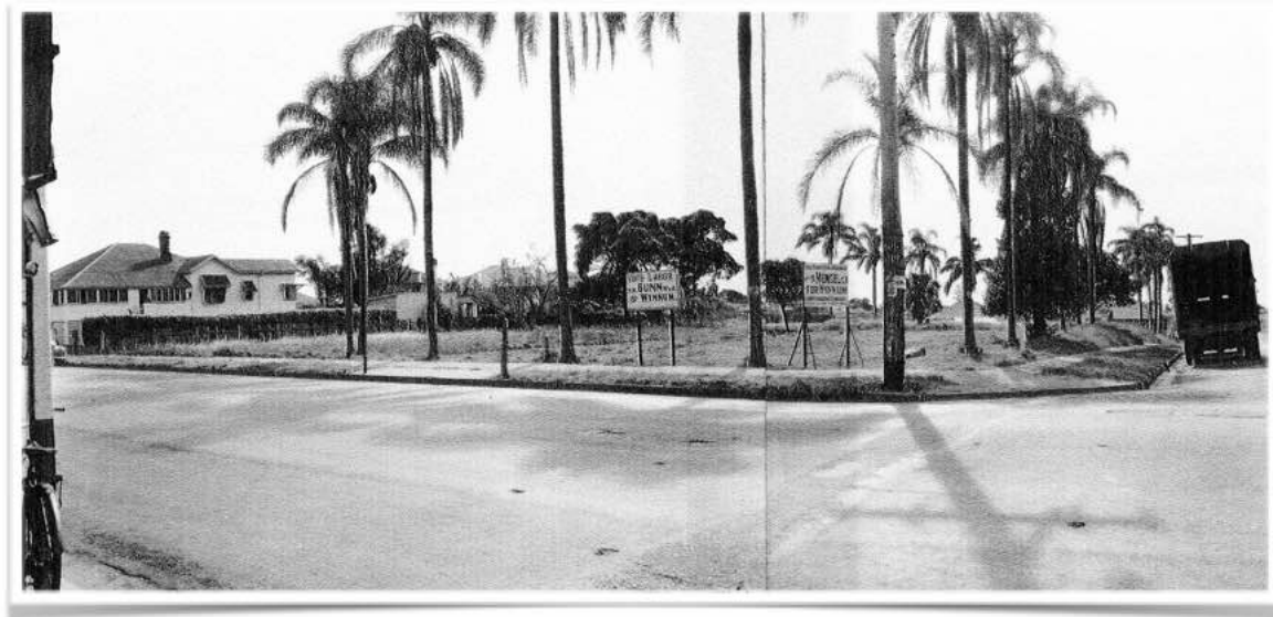
Ingleston Corner at crossing of, Bay Terrace and Charlotte Street. 1947 – 1955
