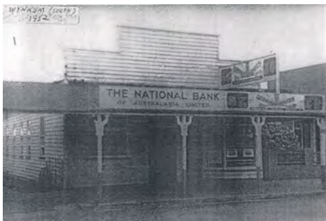
National Bank Bay Terrace 1952 now a 2 storied dental building
