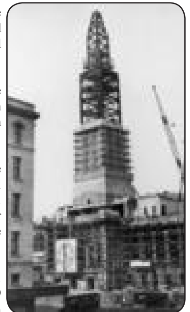
Construction of the tower 1928.
