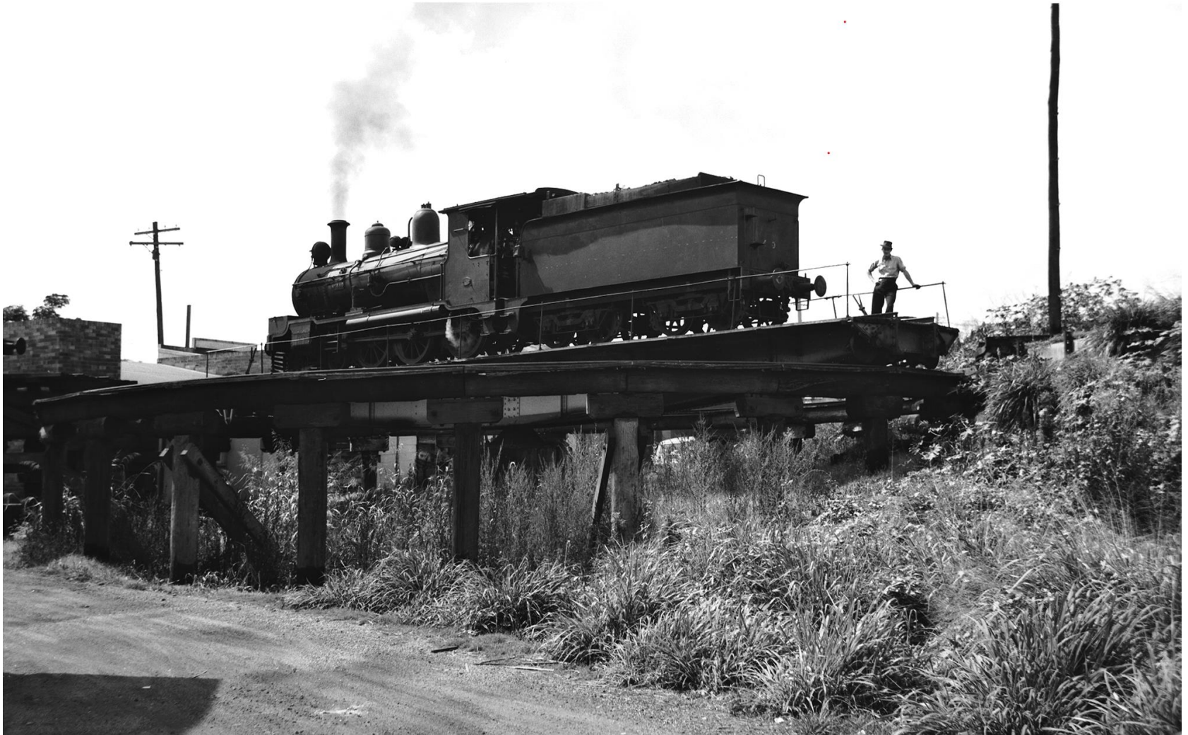
The Wooloongabba depot in 1967 and turntable. The turntable itself was unique in Queensland in that it was of elevated construction. Courtesy: Eric Marggraf/ QR Historical Collection
