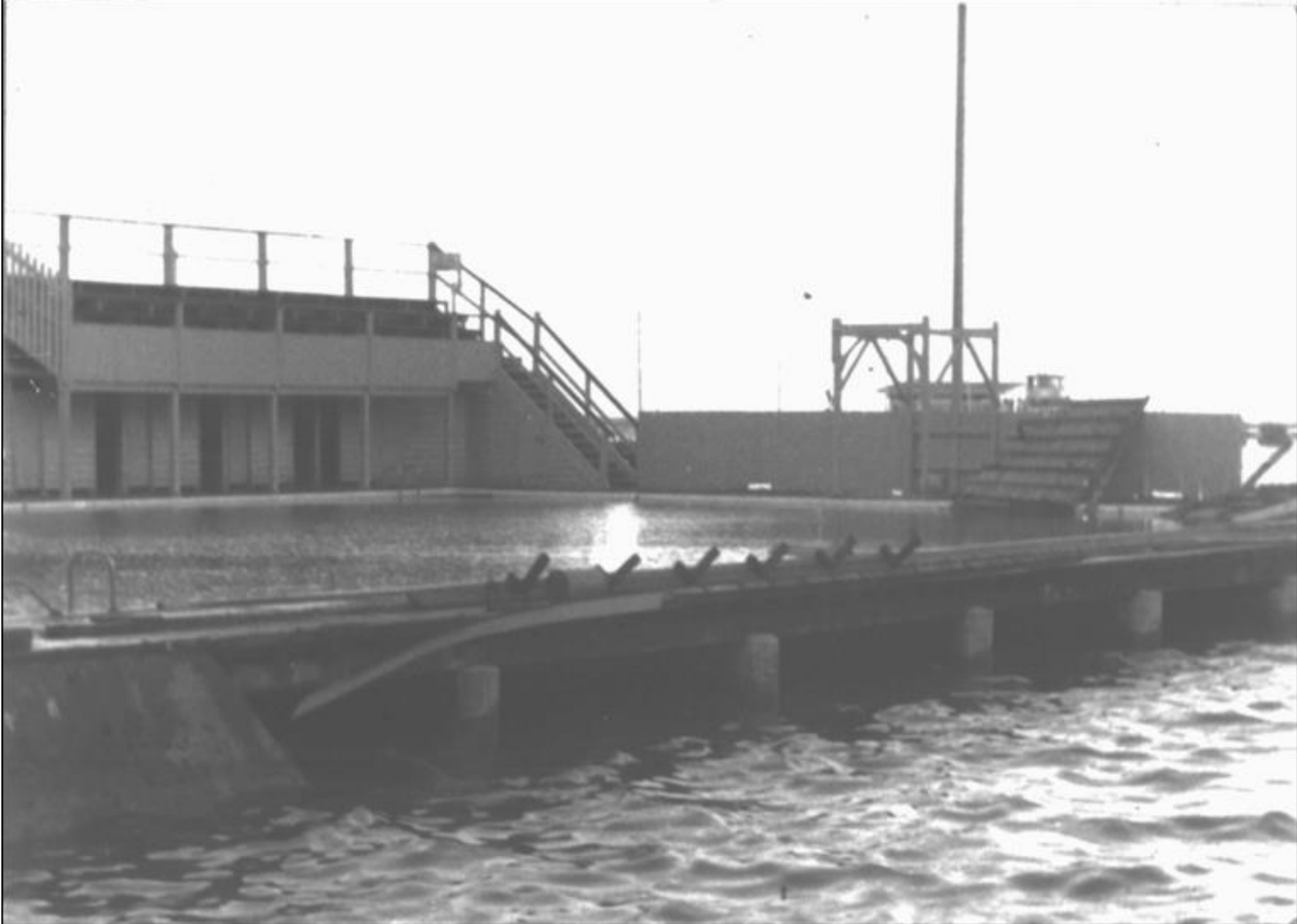
Manly 1959 - Manly Baths after a savage wind and lightning storm – the sheer power of the wind blew one side of the changing boxes into the pool causing embarrassment to a young lady within – this storm caused damage throughout Manly and also to the Manly Hotel
