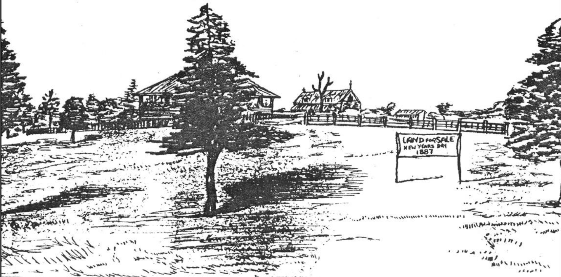
Manly – 1887 Photo No 15 Land Sale - etching taken from a brochure produced for the 1887 sale of more Manly Estate blocks by Arthur Martin & Co auctioneers – to encourage attendance of many buyers, free passage to Manly from Brisbane by the steamer “Kate” was offered plus a first-class luncheon, also free light refreshments were supplied.
