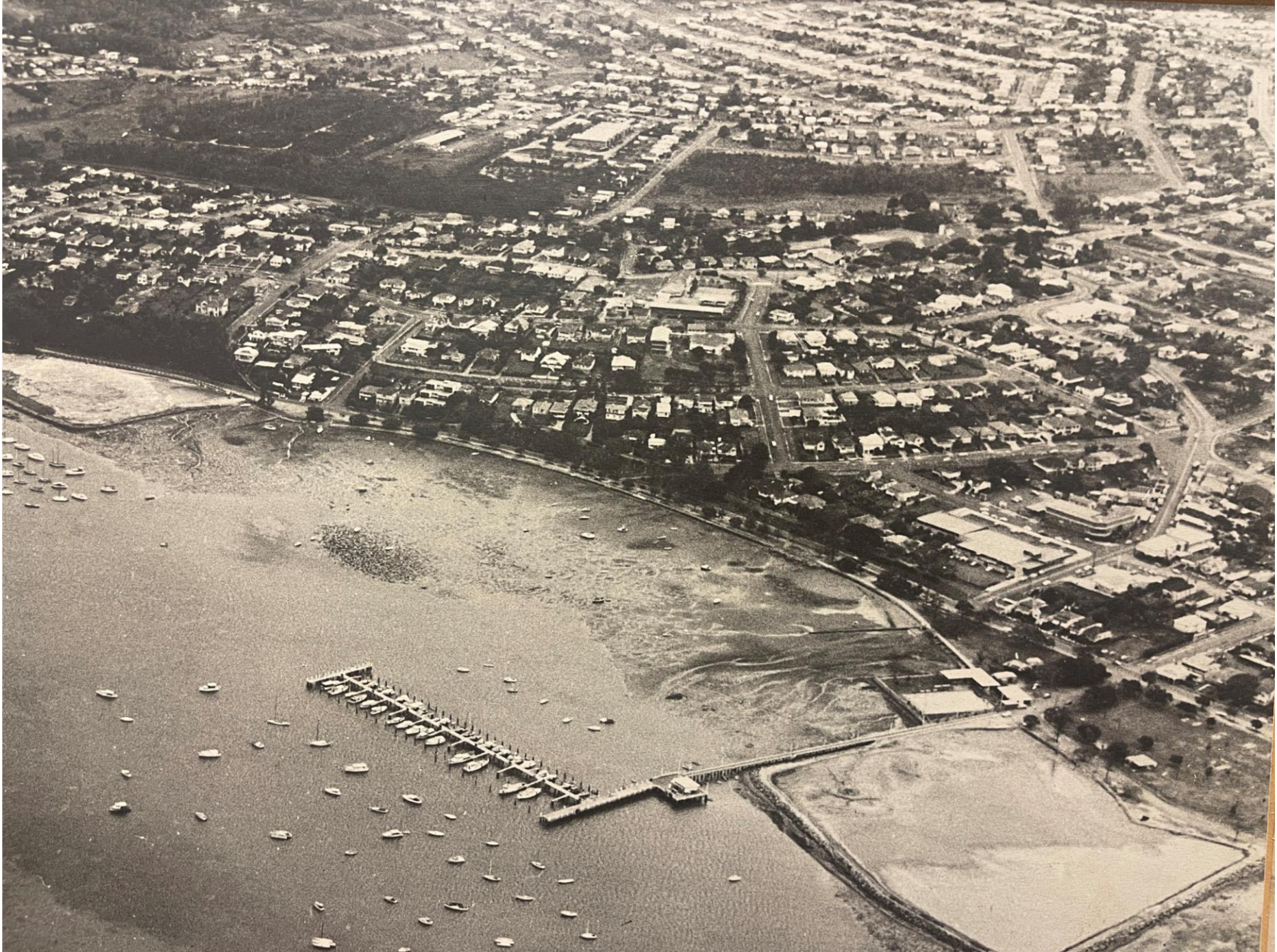
Manly Harbour 1977. The Manly pool can be seen. The area being filled will become the Manly Harbour Boat Club and Moreton Bay Trailer Boat Club.
