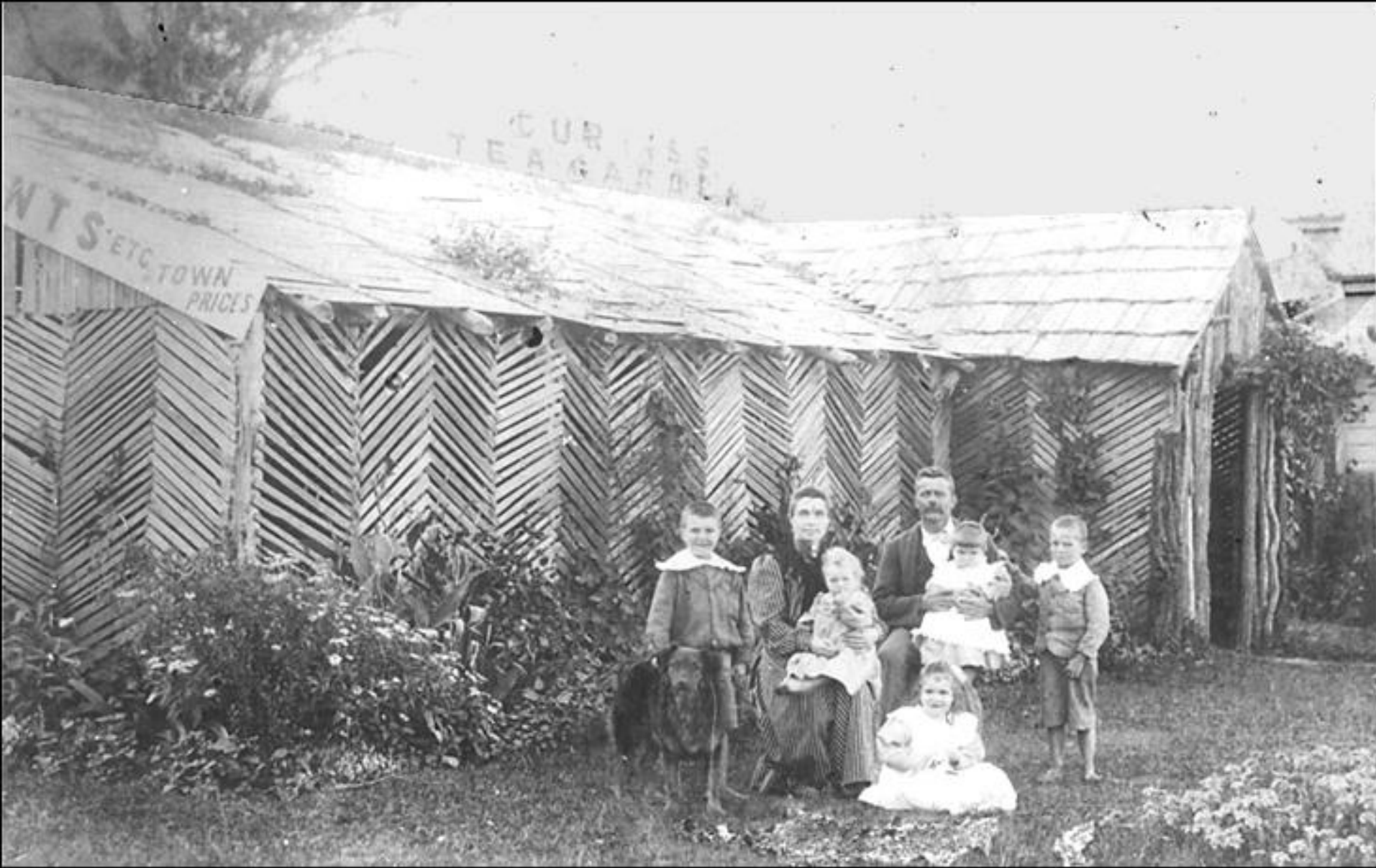
Manly Characters – Traders - The Curtis family posing in front of their Manly tea rooms – Brisbane visitors who alighted at Manly Railway station took the route to the beachfront down Cambridge Parade past all the quaint shops – like the scones and cakes the structure of the tea rooms were all home made – saplings would have been cut with an axe from the bush then carted by horse and cart to erect this building – even the roof is made of shingles of wood.
