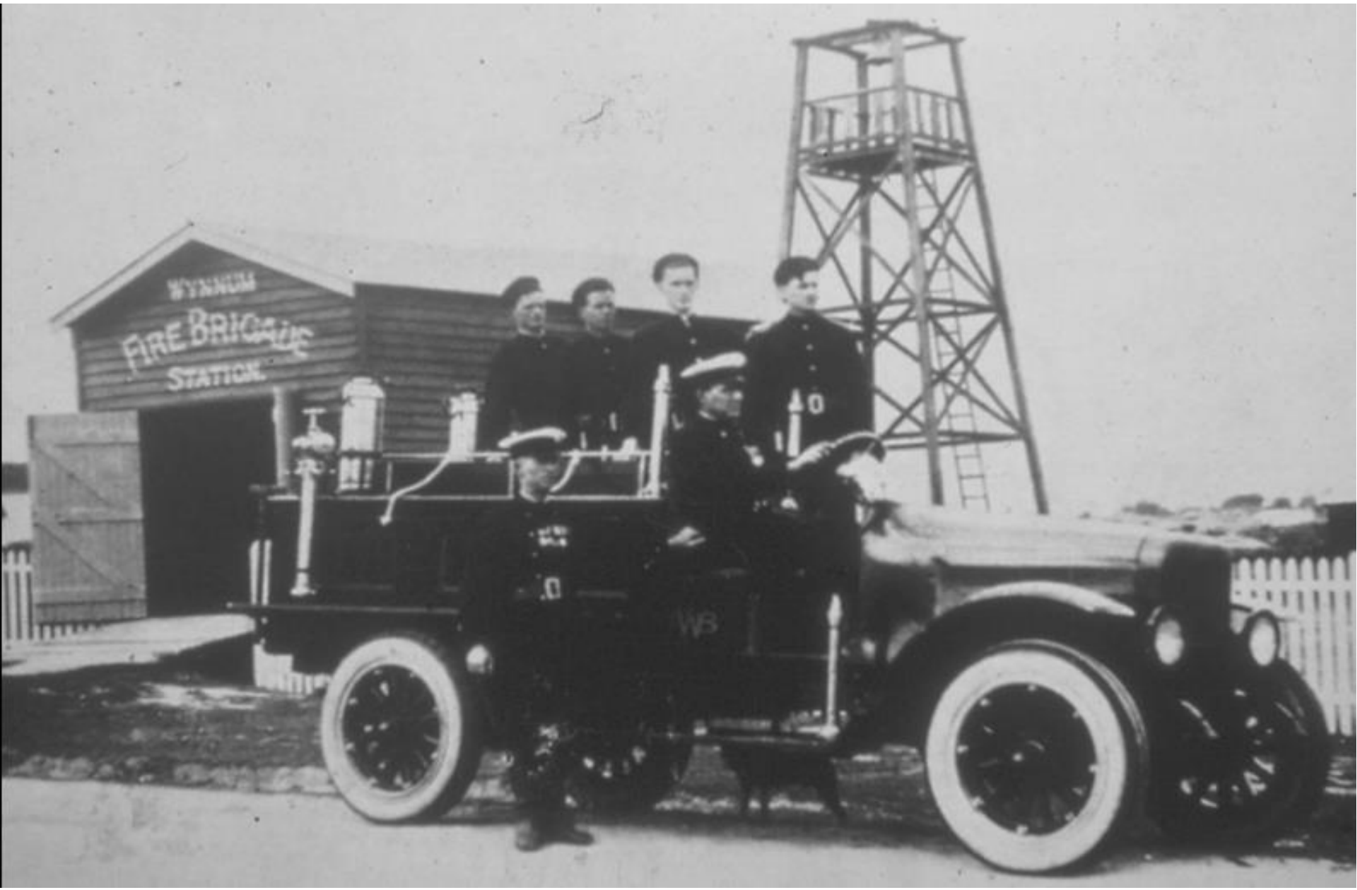
Wynnum – 1922 Photo No 51 Services – Fire - Mountjoy Terrace – at head of Wolsey Parade – following the gradual installation of a town water supply the district could think of establishing a Fire Brigade Unit – this first fire station was built and opened on 25 August 1921 – this photo of 1922 shows the fire brigade Captain and other volunteer firemen proudly posing for the photographer with the new engine Myrtle Beitz, August 2005
