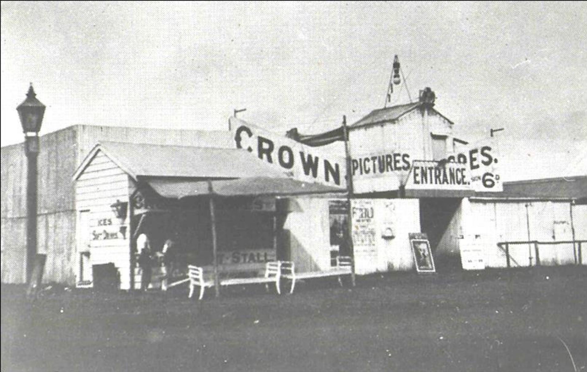
Wynnun – 1915 Photo No 60 Beachfront - Theatres - Buildings – Entertainment –corner Esplanade and Florence Street Wynnun (Central) South – High walls of galvanized iron surrounded this Crown Theatre without a roof - in time, a framework was erected to allow tarpaulins to be pulled across in bad weather - entrance fee 6d. in the 1920s - outside gas light and hitching rail are evident of the time – with many improvements, this theatre became the Imperial under the ownership of Mr Geraghty in 1930.
