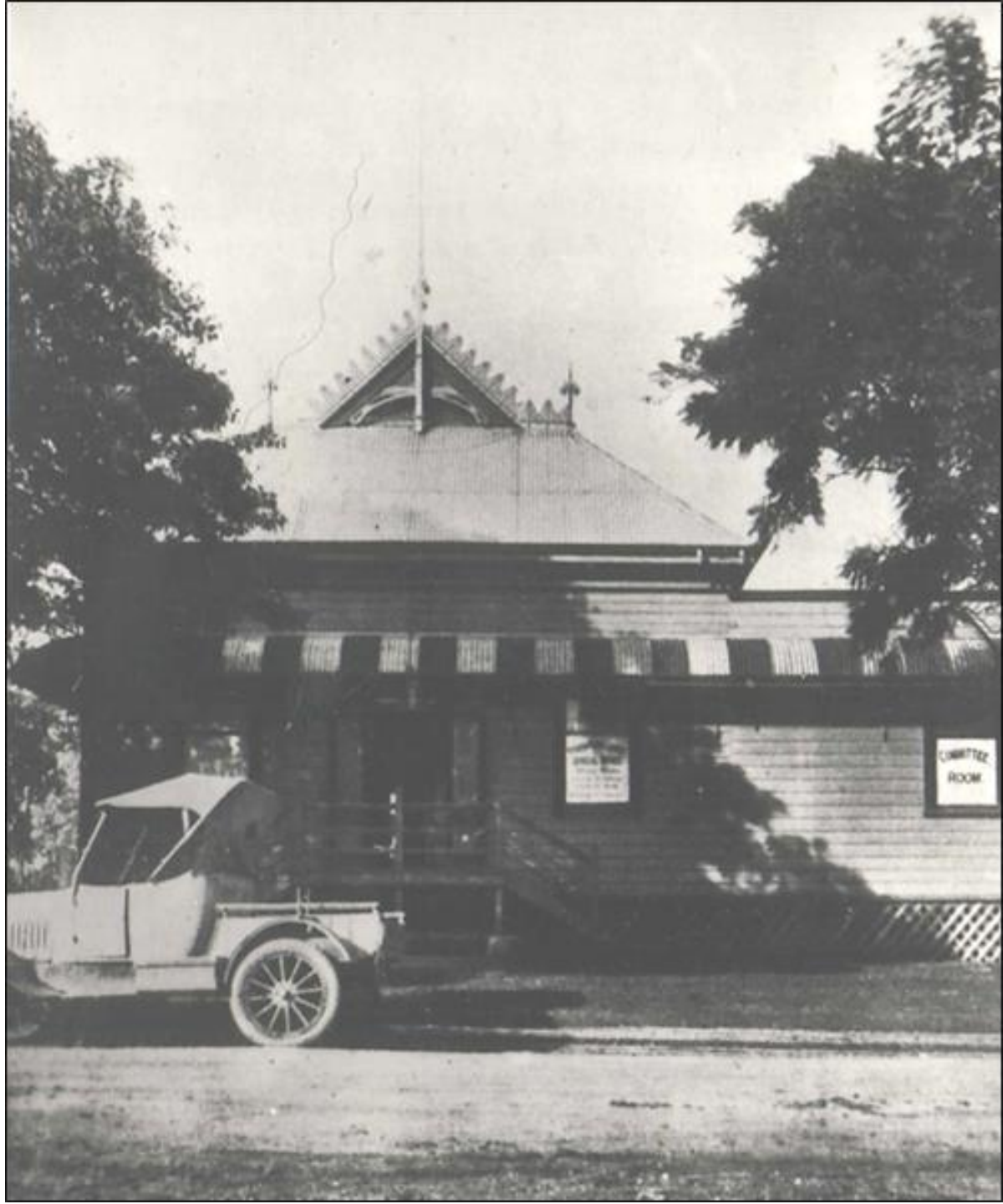
This photo was taken in 1921 of the Shire Hall situated in Tingal Road Wynnun; celebrations in the form of a Grand Concert took place for the opening of this Hall on 8 August 1890. The matters relating to local business were conducted in this building prior to the district becoming part of the Brisbane City Council in 1925. By 1977 the Old Town Hall outlived its usefulness and was demolished in 1977 to make way for the Waterloo Bay 50's and Over Centre . The utility in this photo is believed to belong to the photographer.
