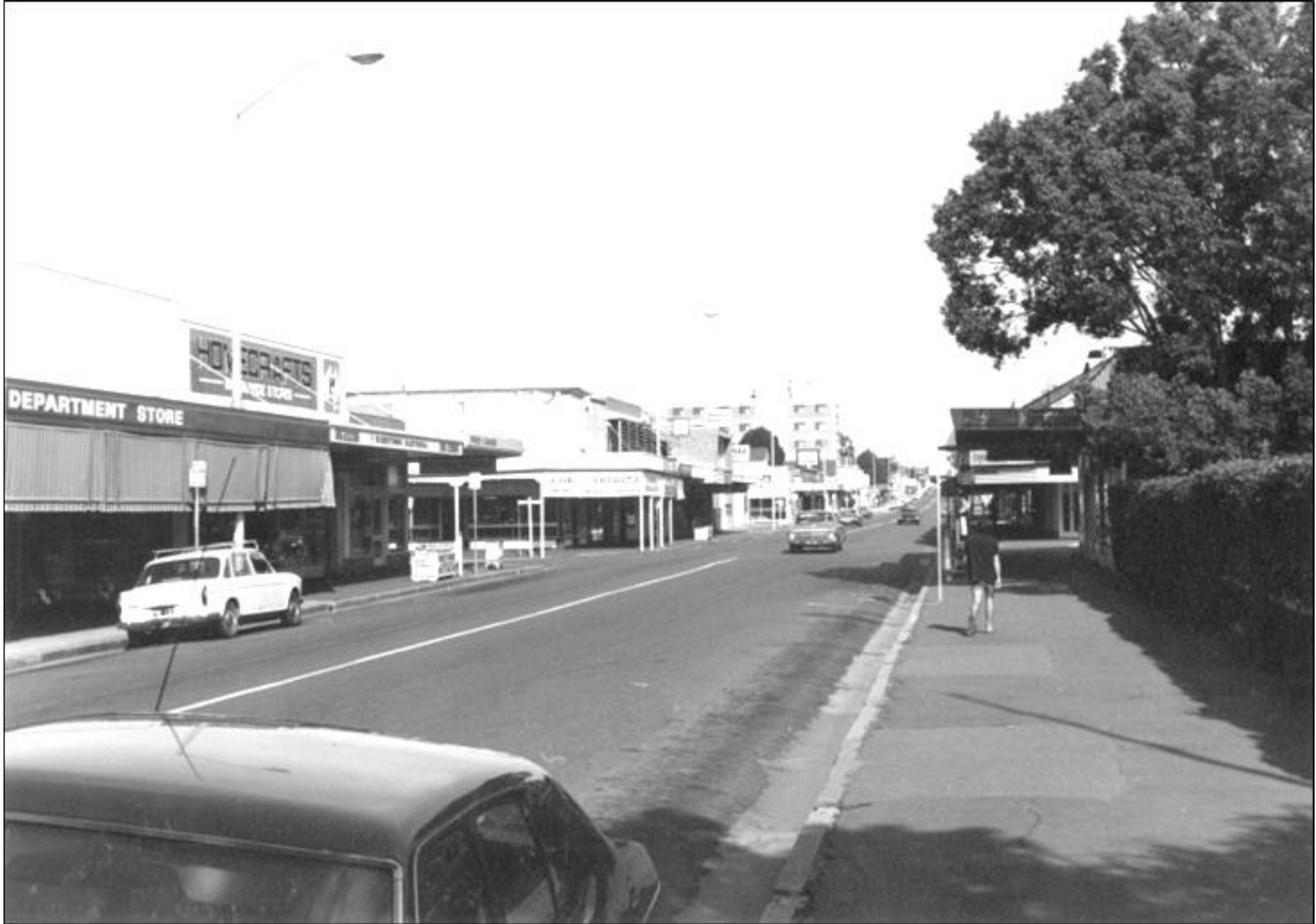
Wynnum – 1978 Photo No 203 Bay Terrace – Shops - Another record of the many times photographed Bay Terrace and Florence Street corner. The hedge, trees, shops and awnings together with Moreton Bay College were removed in 1987 to make way for Franklins shopping complex. Myrtle Beitz, August 2005
