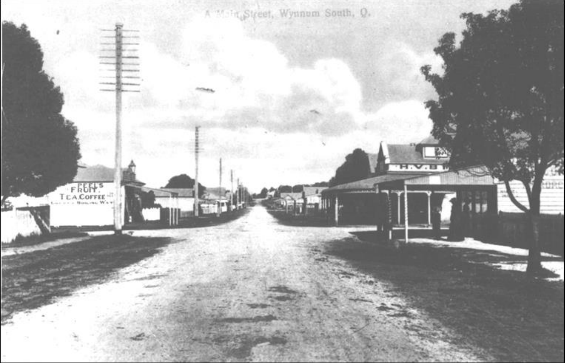
Wynnum— 1920s Photo No 28 Shops - Bay Terrace —looking south from Florence Street corner showing a large increase in the number of telephone lines, supported by 10 cross bars, (so me earlier photos show only 3) - pole to left is supporting a gas light - Peel's fruit and vegetable shop (beach side) is opposite Birchley's store - northern corner on beach side is still a private home - other corner has a butcher's shop under the control of the State Butchers with Samuel Burrows as manager in 1933. The business was sold to Mr Burrows and later to Mr Phillips. A barber's shop was next door – no gutters and grass sidings are shown to the gravel road. See also Photo Nos 1,4,17,23,29,39,32,167 (looking south) Myrtle Beitz, August 2005
