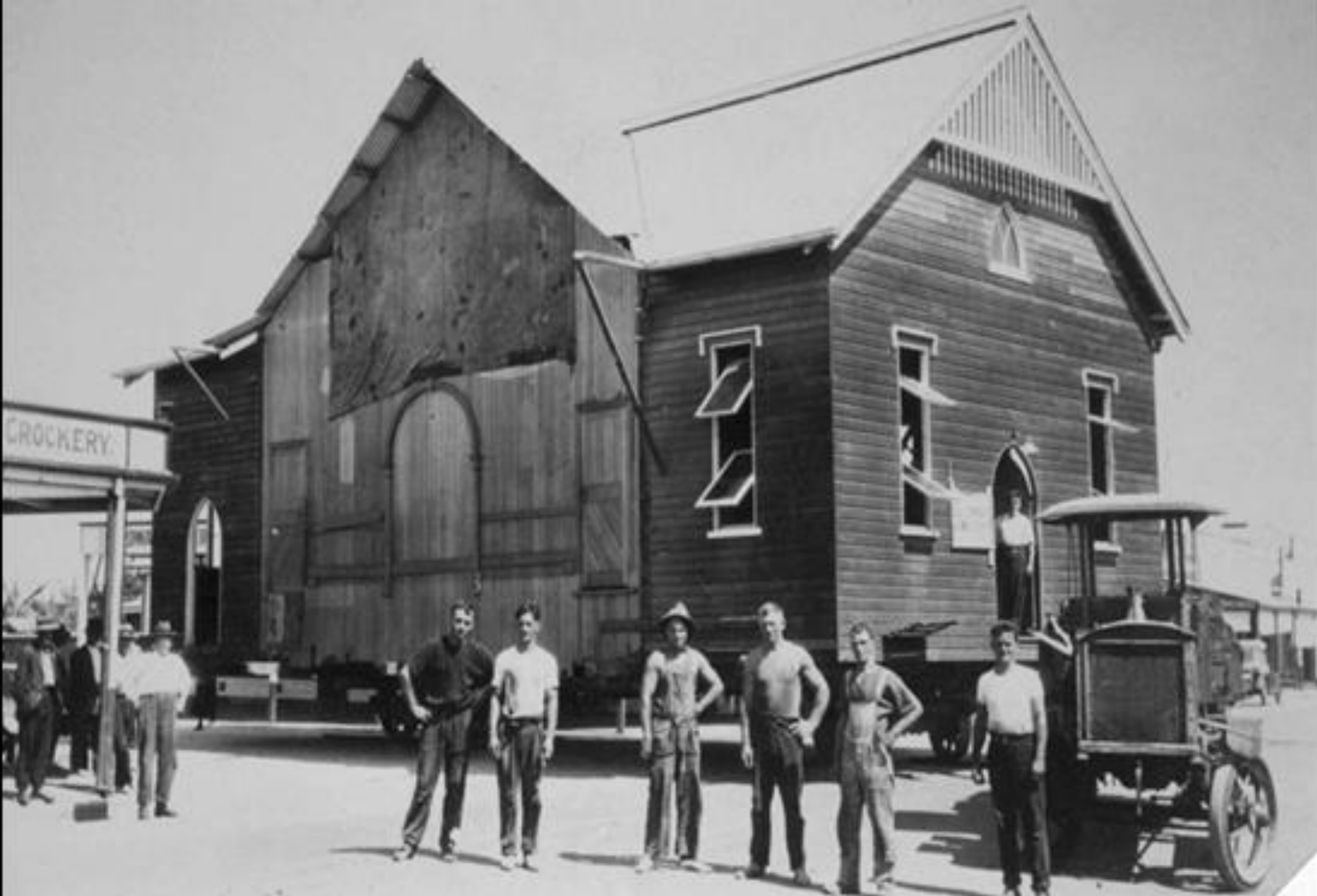
Wynnum – 1930 Photo No 311 Churches - Moving of Baptist Church, turning from Edith Street into Bay Terrace transporting to Corner Clara and Bay Tce, beach and south side. Originally built 1912, was unlined and very small acquiring the name “The Butter Box”, later extended to length affording three to five windows and adding a vestry and small hall – Mr & Mrs Humphreys donated the land for it to be removed to Bay and Edith - shifted in two parts. Myrtle Beitz, August 2004
